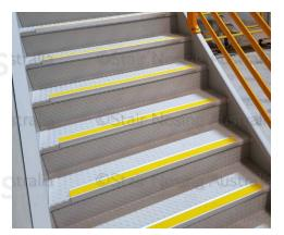
Start by thoroughly cleaning the checker plate surface to remove any dirt, grease, or debris that might interfere with adhesion. This step is crucial, as a clean surface ensures maximum contact between the adhesive and the stair nosing.
